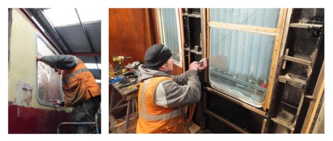
Alan Hardaker is pictured (above) fitting the new clear window to the entrance vestibule. Since these pictures were taken much of the wall and ceiling panelling has been fitted.
