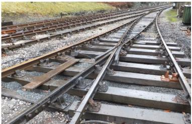
The John Fowler & Co. team are also finishing off the replacement of rail sections and sleepers under the point for the diverging tracks either side of Haverthwaite cattle dock adjacent to the loco preparation area. (Photo left)
