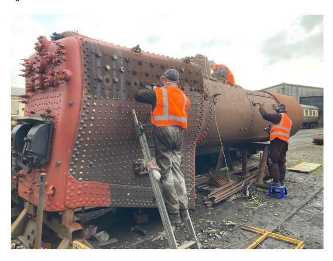
All but the new lower barrel plates are now complete as can be seen in the photo below.
