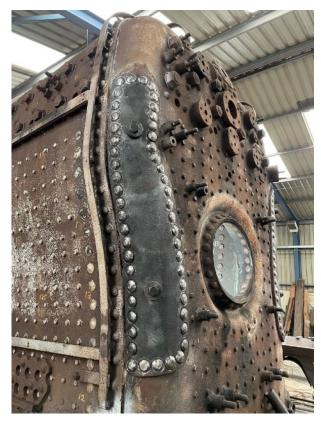
Other than the fitting of plugs, assembly of both of the firebox back shoulder doubler plates is now complete - as can be seen in the photo (left).
