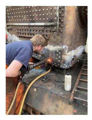
Replacement of worn inner firebox patch screws on the tubeplate flange has been completed.
