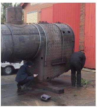
Whilst the boiler is out of the frames Fred Jones is busy removing the years of accumulated ash and coal dust from the footplate area and is cleaning up the inside of the frames ready for a coat of paint.
