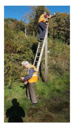
Volunteer Keith Brewer supported by Fred Jones are carrying out a programme of work to repair the telegraph route between Haverthwaite and Lakeside. This involves replacement of many pole cross arms and sections of wire. They can be seen at work (photo left) near Newby Bridge. The new path near Lakeside has also led to the need to move the routing of the telegraph cabling.
