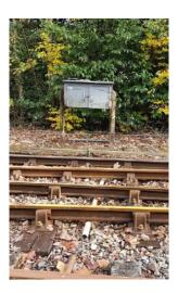
Also at Lakeside, Cliff is preparing to reconnect the 16A points leading to what was the long carriage siding in BR days. This can be seen on the top right of the photo (below right). These points have been previously clipped in a fixed position for the run round loop with the siding isolated. To reinstate signal box operation, the refurbished rocker arms (photo below left) have been fitted and rodding laid out in preparation for connection of point blade actuation and interlocking.
