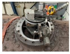
The top feed flange face can be seen during machining (photo above right). All boiler mount faces have now been machined and all mounting studs fitted.
