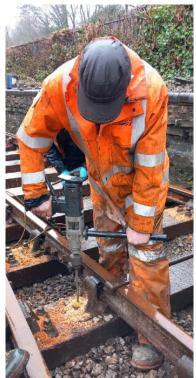
By the last week of March all the new timbers and track were in place with the final chairs attached. Photo (left) shows Alistair Colquhoun from John Fowler & Co. drilling the timbers. Photo (below) shows L&HR operations staff as they get close to task completion. Just the re-ballasting was required to finish the job off.
