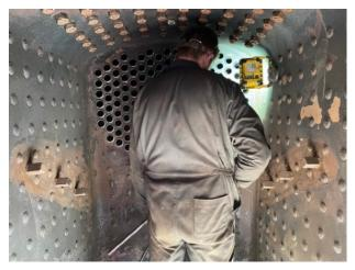
The boiler has subsequently been successfully hydraulic tested (in the presence of the boiler inspector). The steam test is anticipated before the end of April
