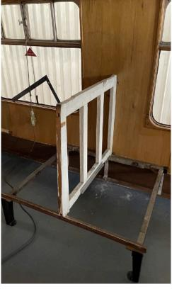
The lower woodwork is in place and this allows the steam heating pipes to be re-fitted. The first seat frames are also being installed. Photos (above and left).
