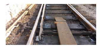
Cliff has also done adjustments to improve the crank action on the Lakeside ground frame points as seen on the left of the photo (left). This has given them a smoother operation.
